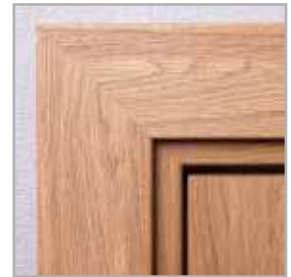
standard interconnection of architraves at the 45° angle
