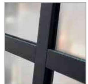
glazing bars glued onto the glass
